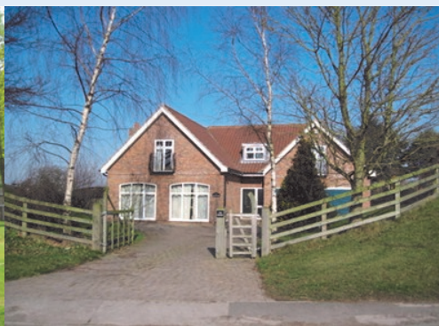
Bungalow built on the old railway trackbed.
