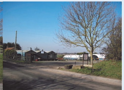
Disused nursery buildings.
