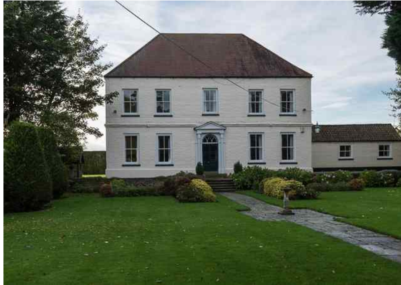
Manor House Farmhouse, Strensall
