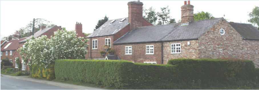
Eighteenth and nineteenth century cottages and outbuildings, 17 to 21 Church Lane
