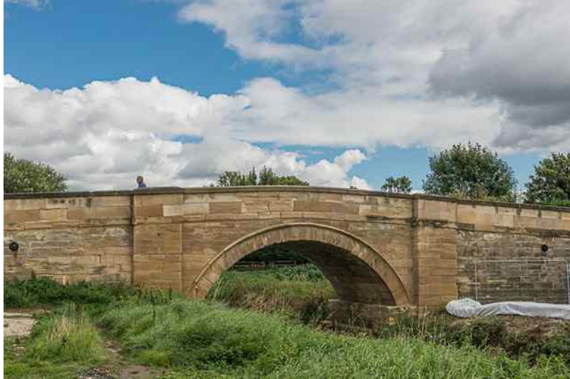
Strensall Bridge - John Carr's Bridge
